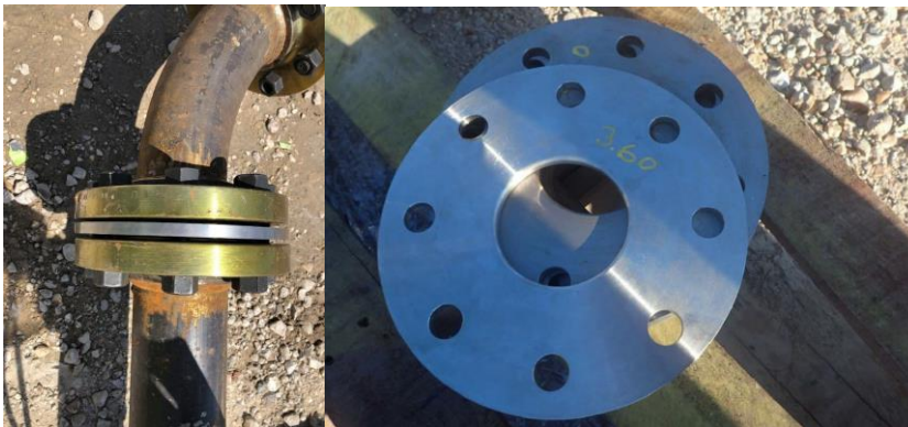
Figure 3 Machined Rings Inserted Between Flanges
