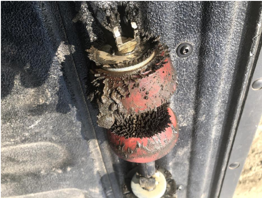
Figure 2 Debris on Magnets of Cleaning Pig
